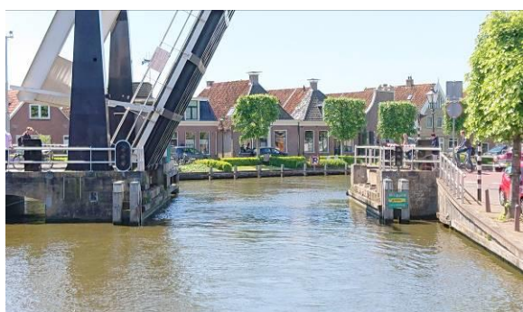
Lifting Bridge at IJlst
