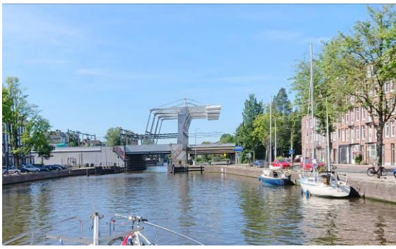
Railway bridge for the night convoy
