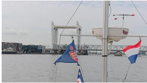
Dordrecht lifting railway bridge
